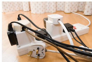
Electrical overloading hazard
