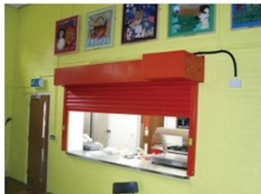
Fire resisting roller shutter
